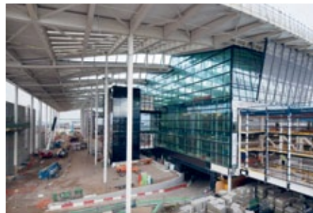
Top: The installation process, 2014. Above: A view of the forecourt area as Terminal 2A is constructed, 2012
