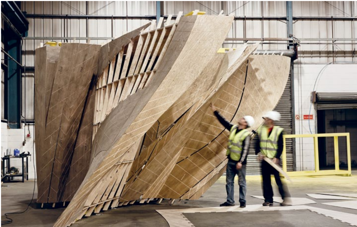
Above: Fabricators with a section of Slipstream under construction at CSI factory in Hull
